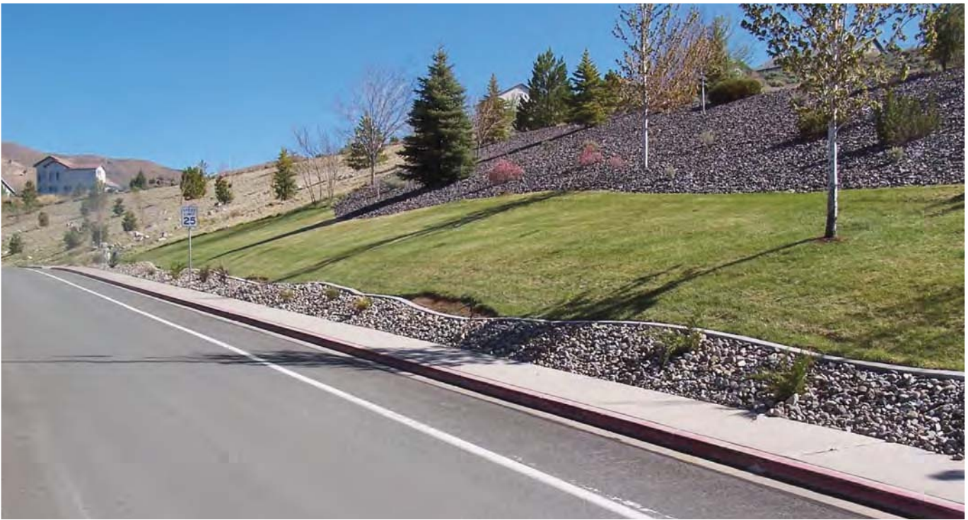
Figure 2: Landscape xeriscape buffer to reduce water runoff in catch basins.
